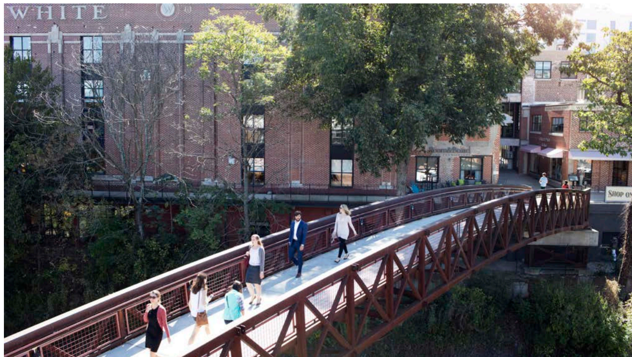
Example of a well-designed pedestrian bridge at White Provisions in Atlanta, GA
